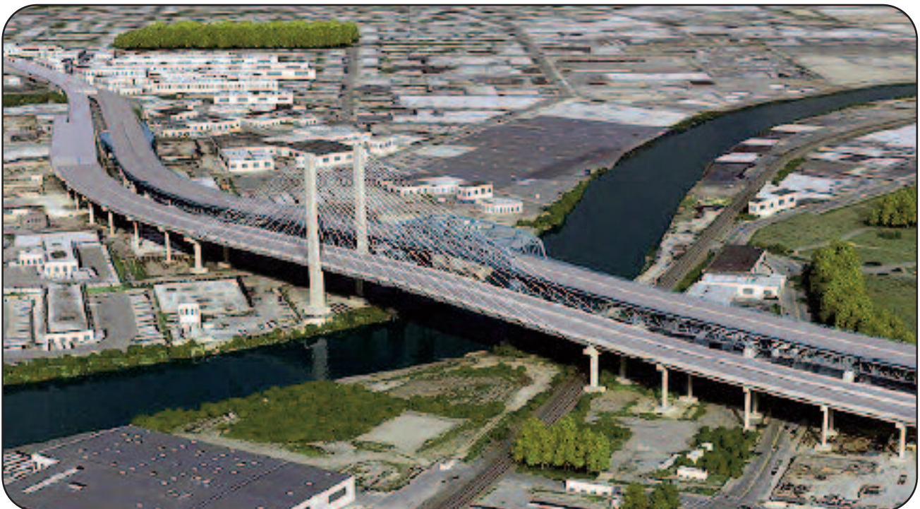
New Queens-bound bridge built beside existing bridge.
