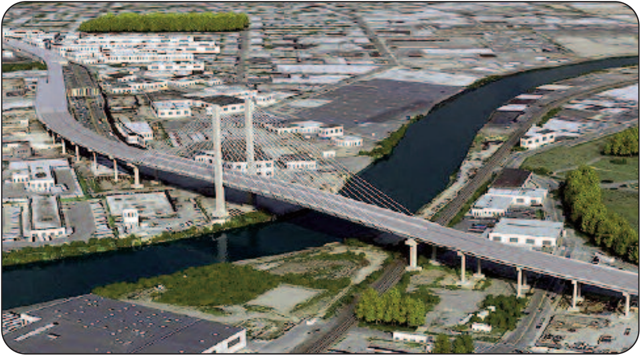
Removal of existing bridge, making way for new Brooklyn-bound bridge. All traffic is shifted to new bridge, until Brooklyn-bound bridge is constructed in Phase 2.
