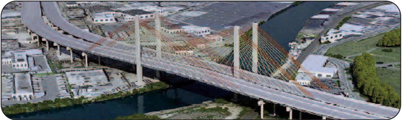
New Brooklyn-bound bridge constructed beside new Queens-bound bridge.
